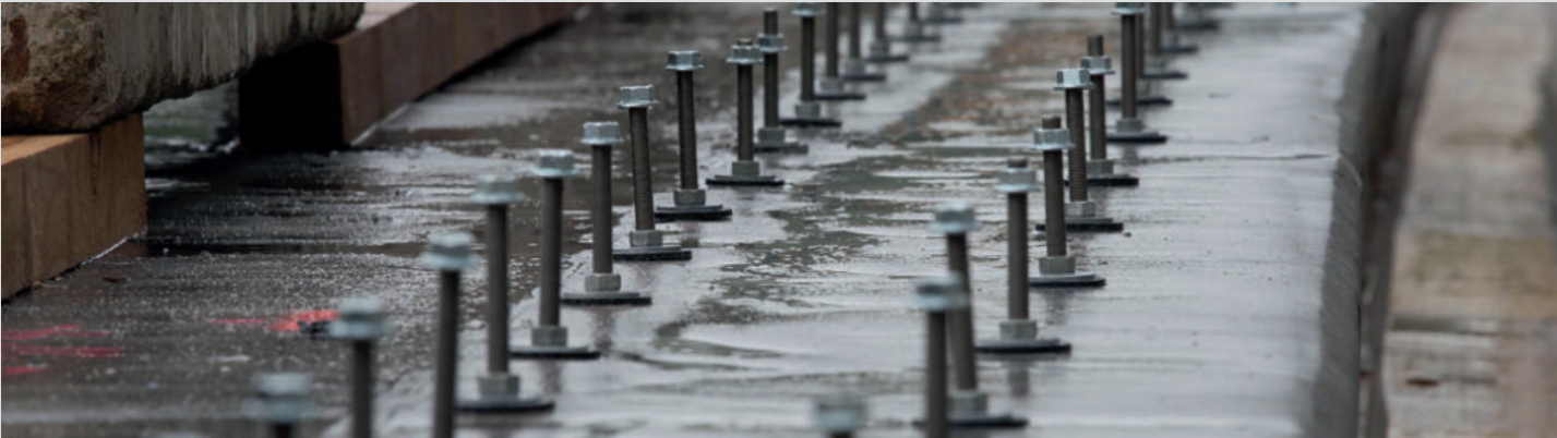
Bridge edge beam fixing
